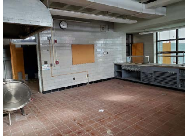
Photo 14: View of kitchen (former) within the classroom wing addition to the building on the TP.
