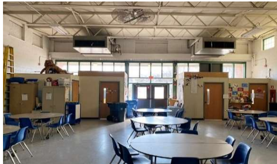
Temporary rooms added in the Cafeteria.
