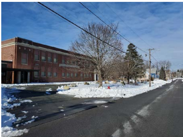
Photo 23: View north-northeast from Old Street of building on the TP.
