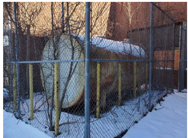
Photo 18: View southeast of 6,000-gallon AST at original / classroom wing addition to building on TP.
